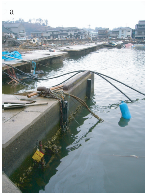
Fig. 3 State of the wharf after the disaster. The wharf fixed the wave height meter was destroyed over tens of meters (a). The trace of tsunami was found near the window of the second floor (b).
